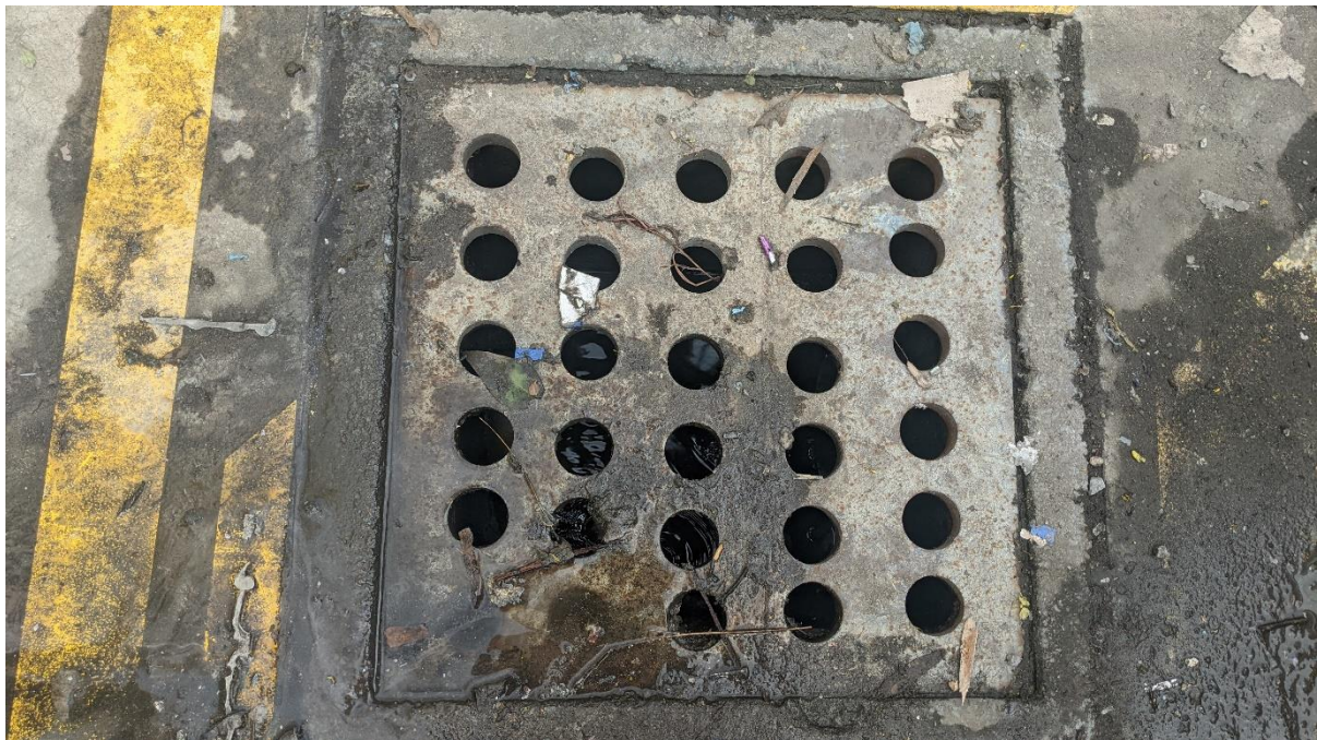
Photo 11 – Stormwater pit with no valve or filter bags installed as required by the Site Stormwater Plan
