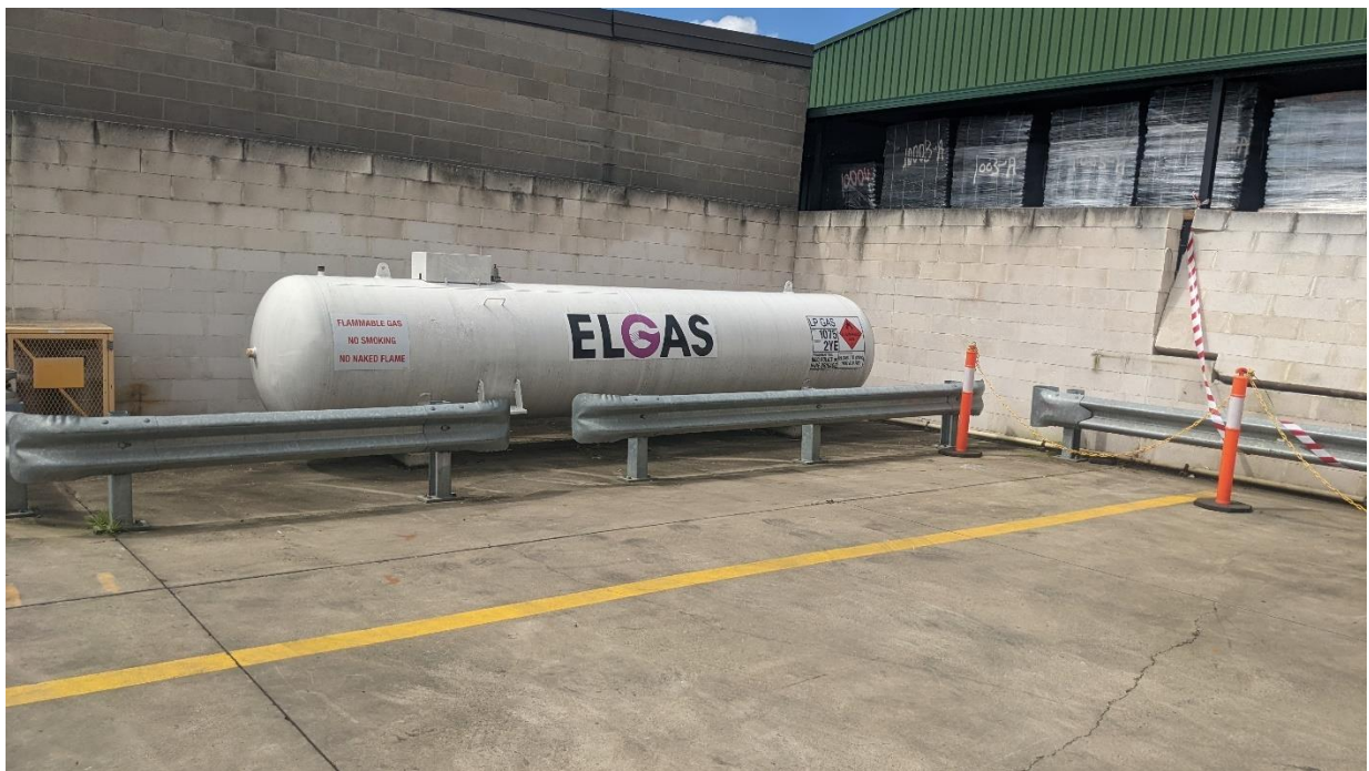
Photo 9 – LPG tank. Yellow exclusion zone line and W-barriers installed.
